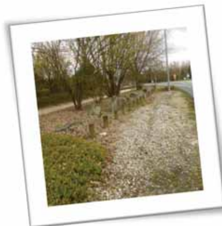
Tranchée drainante, Saint Priest
